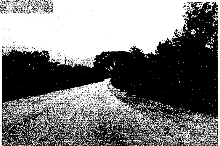
RW7-1 Flooding Section on Route 4063
