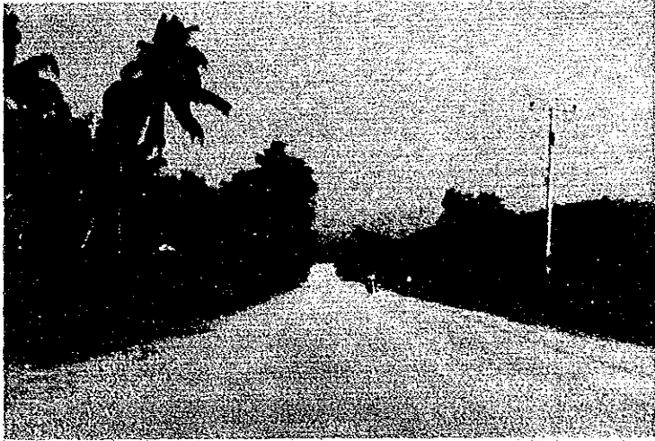
NC-1 Typical View on PWD Road (Laterite Surface Condition)
