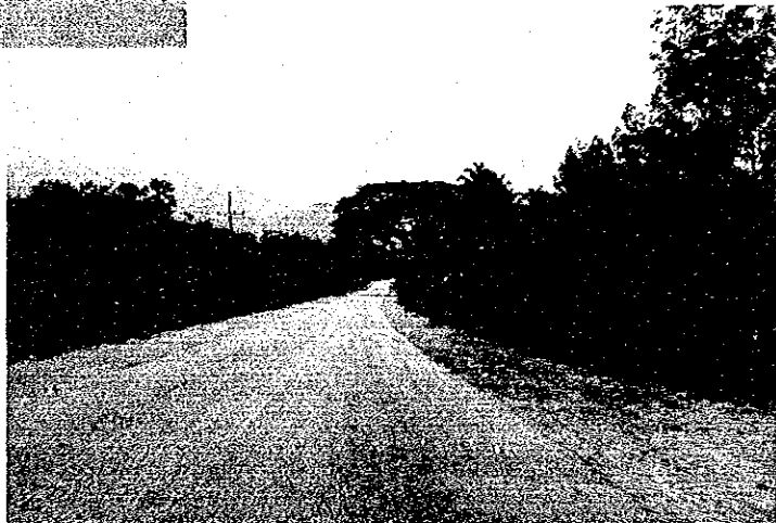
RW7-1 Flooding Section on Route 4063
