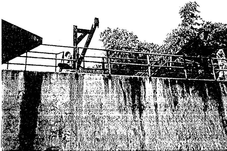
HALAMAN ZOO DUA AERATION TANK AND FINAL SEDIMENTATION TANK
