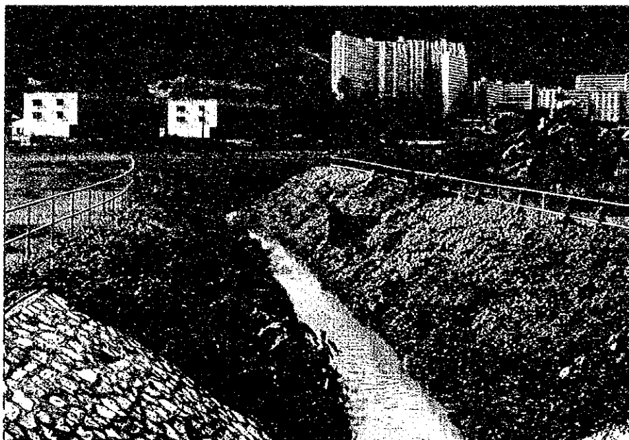
Plate 1: Sungai Dondang Near Proposed Retention Pond A Site.
