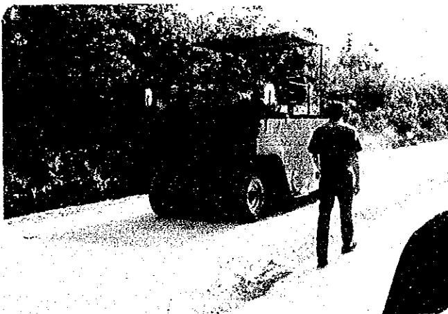
Solidifying subbase course by rubber-tire roller
