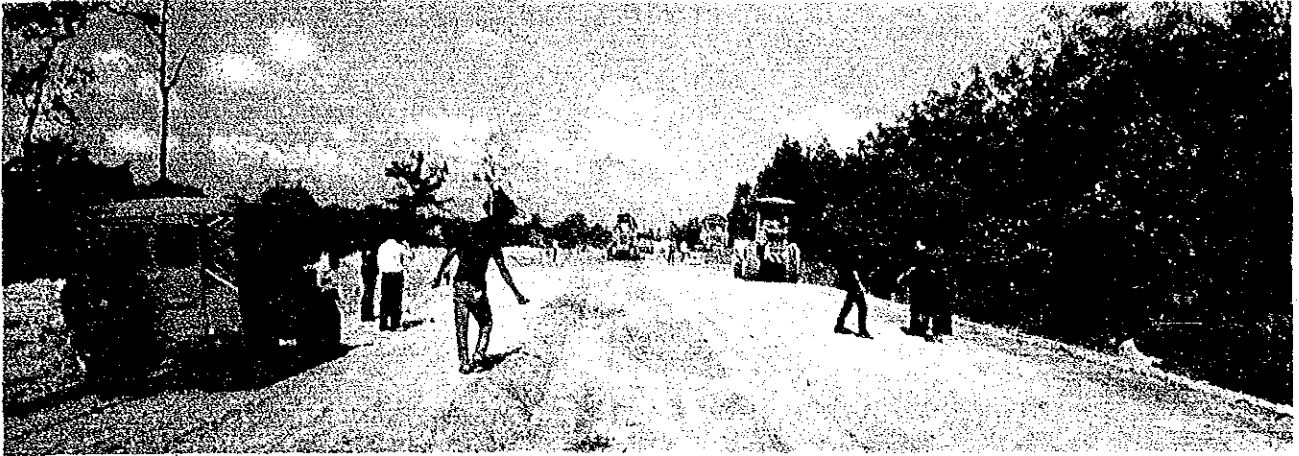
Solidifying and spreading subbase course
