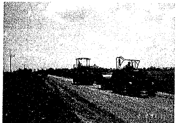
Road construction by rubber-tire roller and vibratory roller
