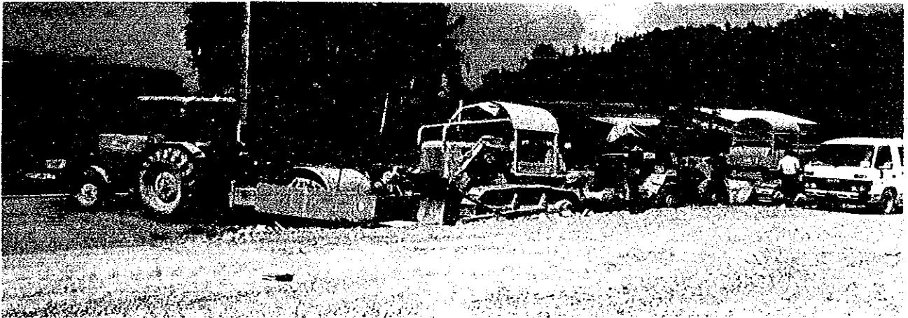
Construction equipment at site
