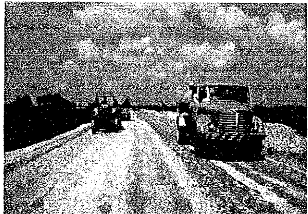
Road construction by water truck
