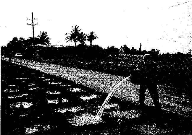
Water curing of hardened concrete
