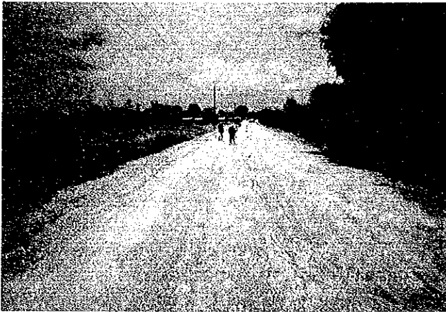
Prepared base course before prime coating
