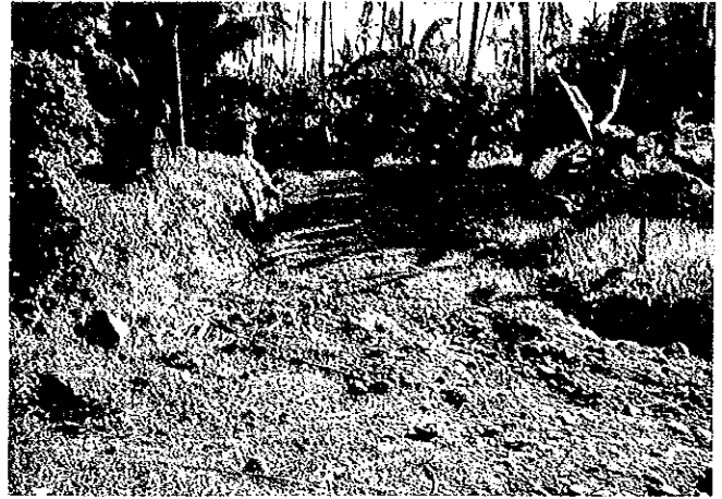
Binuangan-Kidampis Road, Misamis Oriental Gravel road in very bad and narrow section
