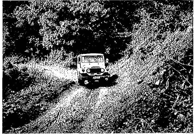
Aringay-San Jose Road, LaUnion At slope failure section
