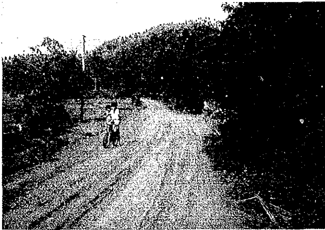
Camalig-Taladong Road, Albay Gravel road in bad condition
