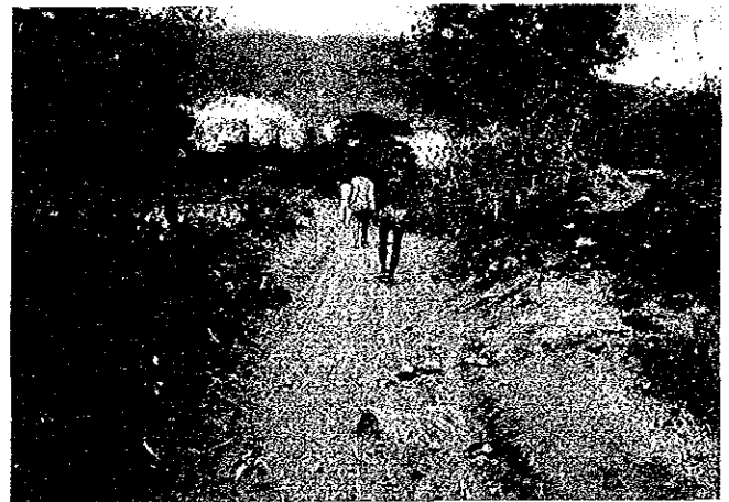
Balac-Balac Road, Antique Earth road impassable for vehicles
