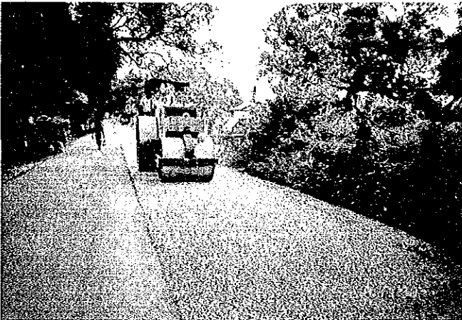
Bituminous penetration macadam, base layer compaction
