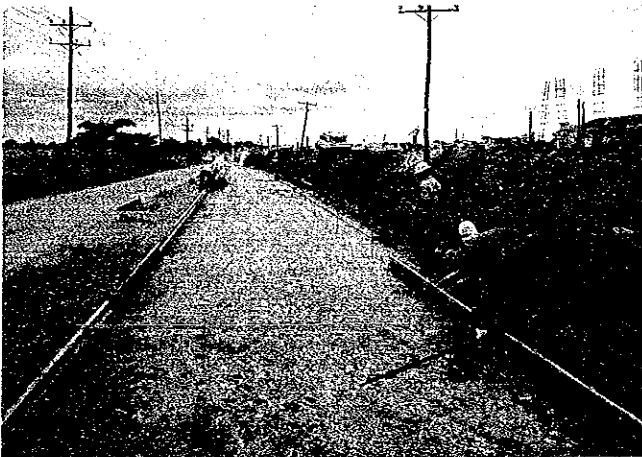
Setting of wooden side forms for portland cement concrete surface course
