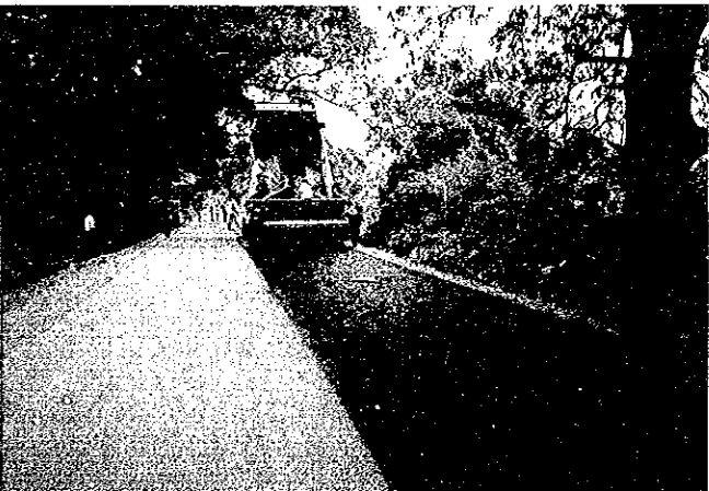
Bituminous penetration macadam, cover aggregate spreading
