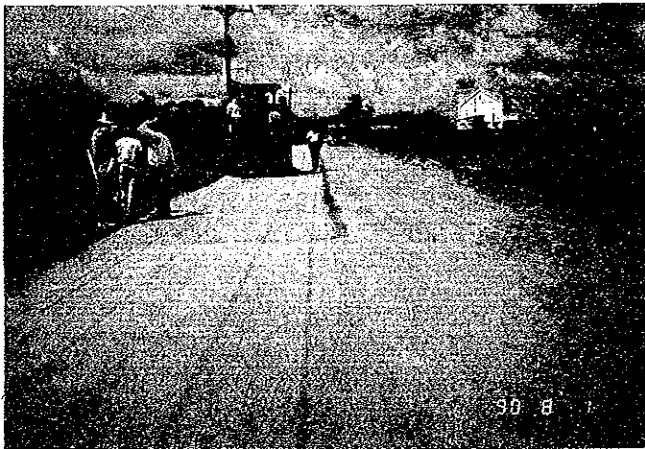
Final rolling of double bituminous surface treatment
