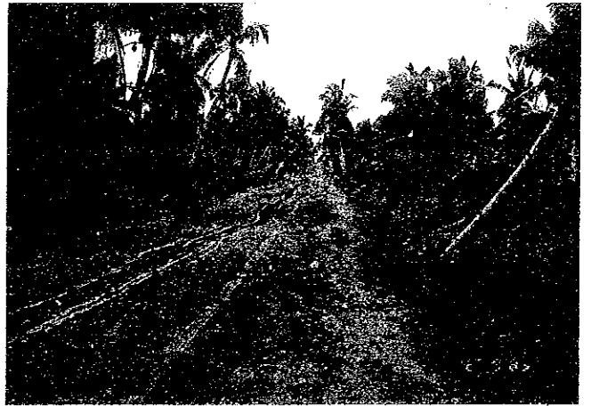
San Juanico-Sohoton Road, Samar Earth road
