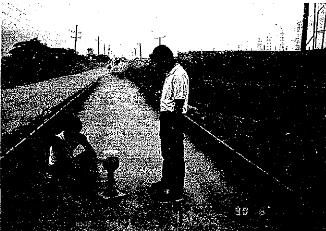
Conducting of field density tests for compacted subbase course
