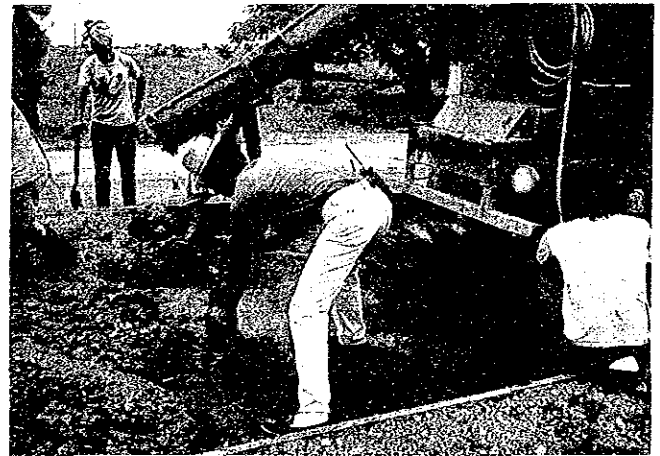
Starting of placement of cement concrete and slump tests
