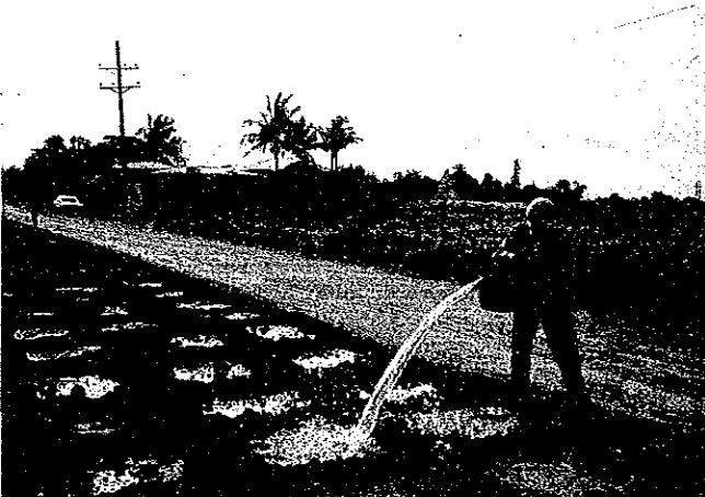
Water curing of hardened concrete
