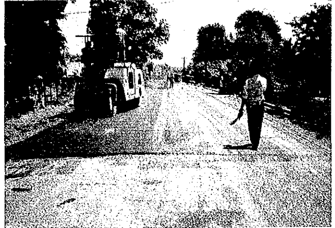
Rolling of asphalt concrete (left) and finished asphalt concrete surface course (right)
