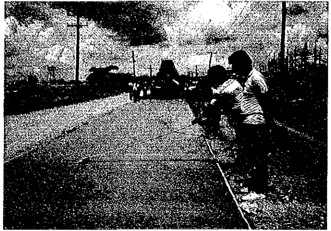
Finishing of cement concrete surface
