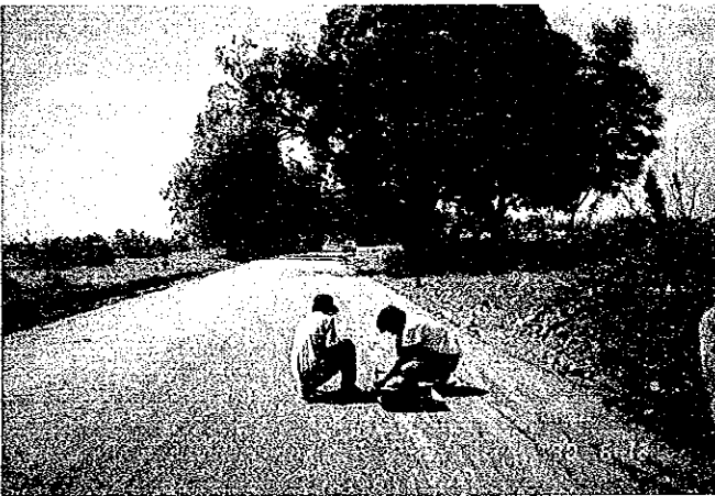
Conducting of field density tests on a prepared subbase course
