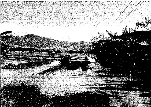
Nueva Ecija-Aurora Road, Nueva Ecija Gravel road at flooded section
