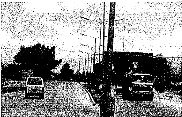
Four-lane highway in rural area with expected congestion in near future
