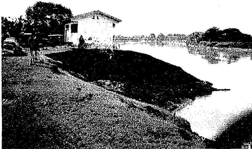
SARIREJO PUMPING STATION (No. 16):
