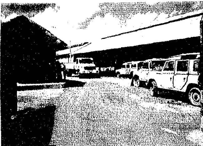
Existing Central Work-shop
