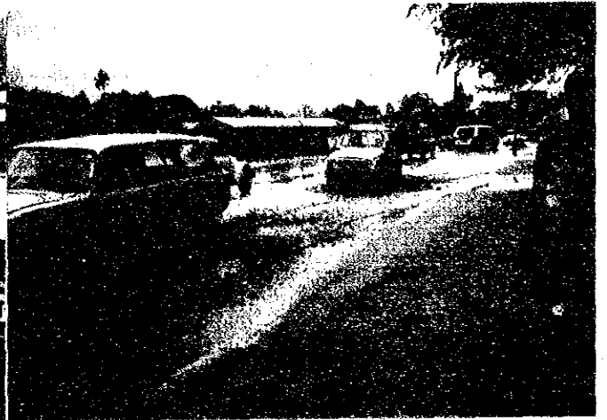
Drainage on Arterial Road
