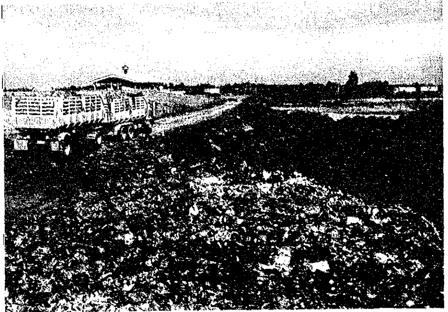
Photo 4 Sanitary landfill by the contractor employed by BMA at Nakhon Pathom Province.
