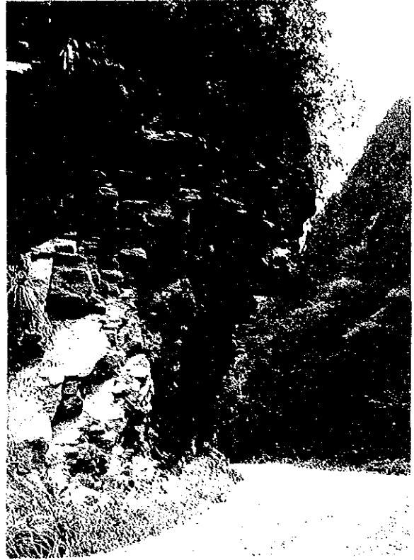
Photo-5 Aspect showing overhang by the road near Puerto León about 35 km from the point of origin. One of the dangerous points for traffic on the study section.
