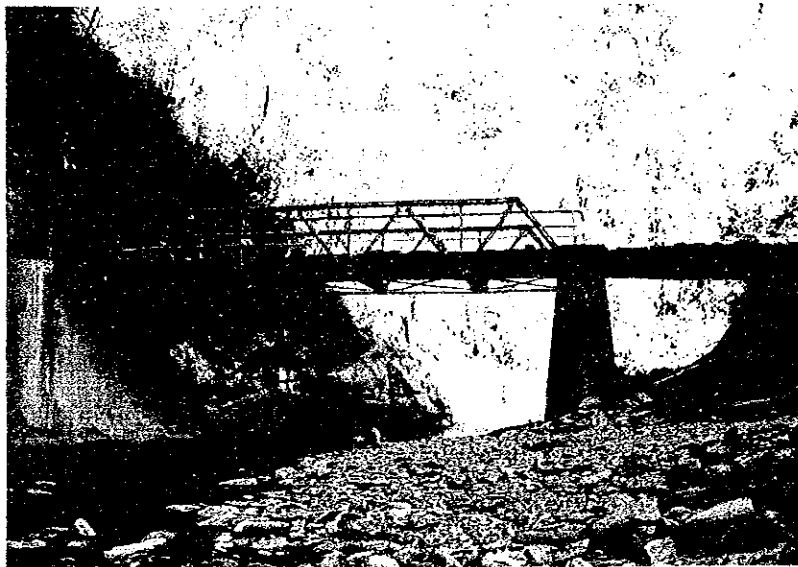
Photo-6 Scene of the present truss bridge near Puerto León. The bridge is old and rotten and wooden slabs have been used in temporary treatment.
