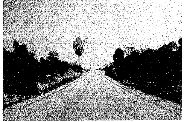
Route 10 after rehabilitation
