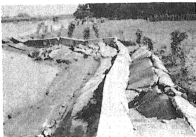
Photo 7.5.2 Damage to a parapet revetment of the Tarlac river
