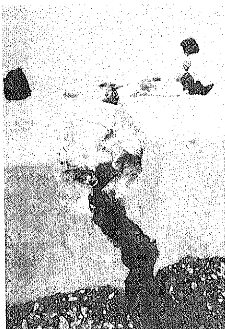
Photo 7.5.3 Damage to a parapet revetment of the Tarlac river
