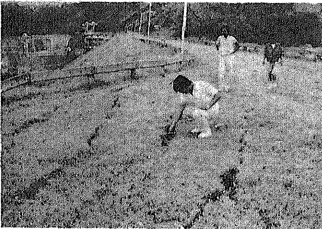
Photo 7.5.42 Cracks on the crest of the Masiway Dam
