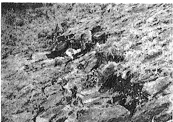
Photo 7.5.21 Sliding of the riprap on the upstream slope-face of the Ambuklao Dam
