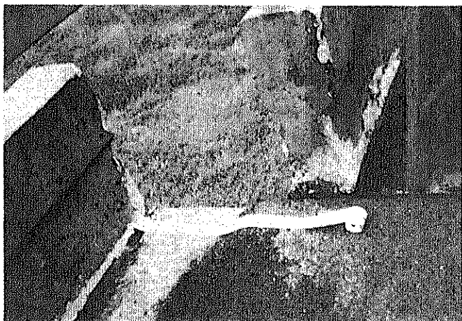
(23-a) Expansion joint slipped out of place by 90cm in direction of bridge axis.
