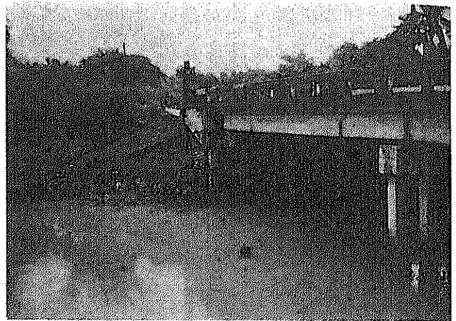
(14-b) Collapsed abutment back-fill (It underwent emergency repair.)
