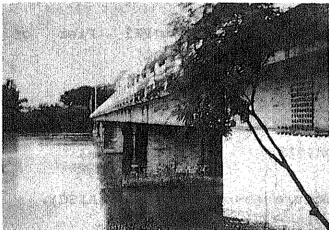
(22-a) Damage to girder ends due to collision between girders. Apparently no damage to piers.
