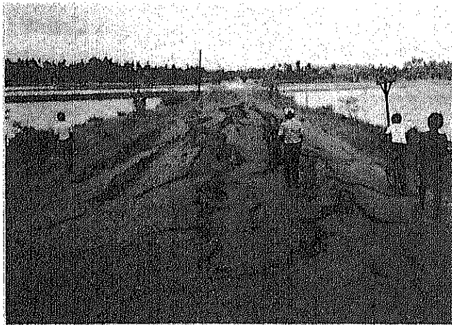
(6-b) Banking in approach settled and moved sideways
