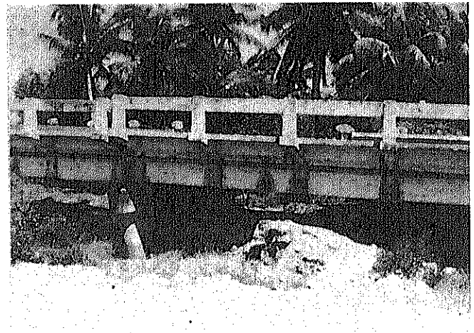
(3-c) Pier tilted by liquefaction
