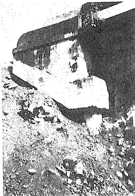
(9-b) Collapsed abutment banking
