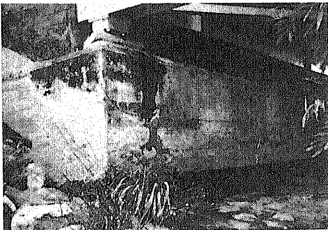
(6-c) Cracks in abutment footing and pile
