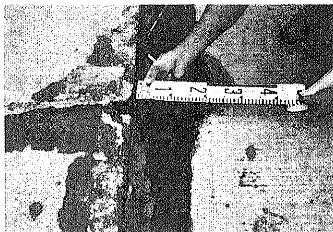
(23-b) Expansion joint opened by 20cm
