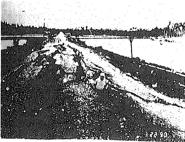
Photo 7.3.45 Crack in bank along No. 313 Line (Courtesy DPHH)
