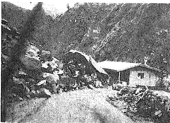
Photo 7.3.59 Masses of collapsed and fallen rocks along the Baguio side of the Kennon Road
