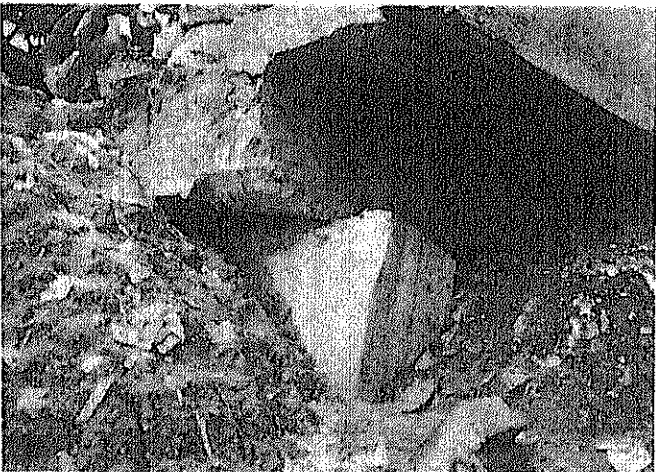
Photo 7.3.41 Left bank abutment of Carmen Bridge; Closer view; side span is pushed out.
