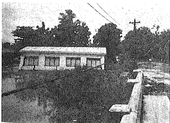
Photo 7.3.35 Road in Barangay Pugo (brought down to a level lower than the water level of the river due to ground sinking.)
