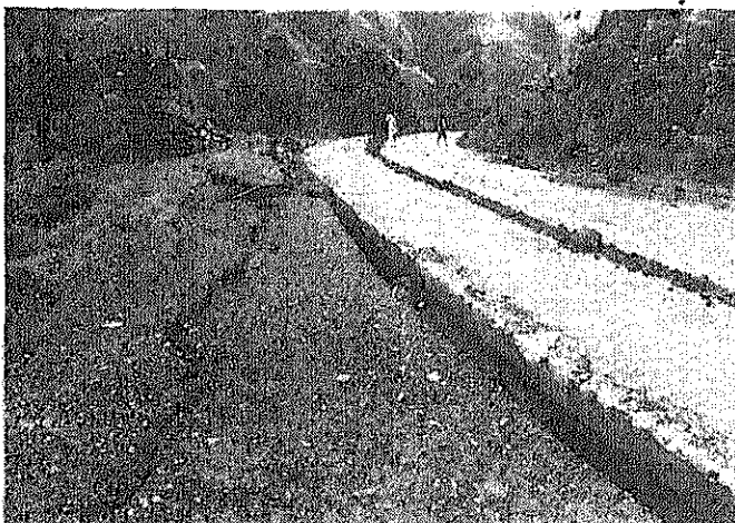
Photo 7.2.15 Opening of the shoulders by the sliding of the banks. (203 km position)
