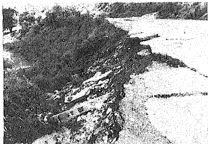
Photo 7.2.16 Collapse of banks. (173 km position)
