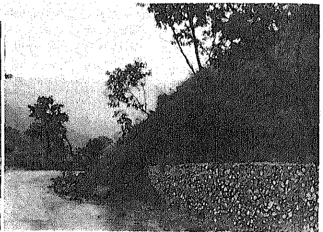
Photo 7.2.19 Small damage at a stone masonry retaining wall (wet masonry with cobbles) as protection of the toe of the cut slope. (201 km position)
