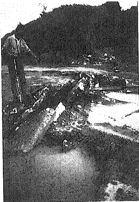
Photo 7.1.7 Earthquake fault crossing the Pan Philippine High Way at KM181. Cracks on the road surface are evident on the fault.
