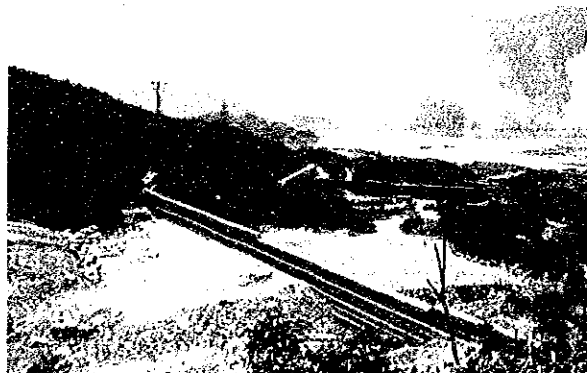
A series of three gabion dams constructed upstream of Ultrafertil.
