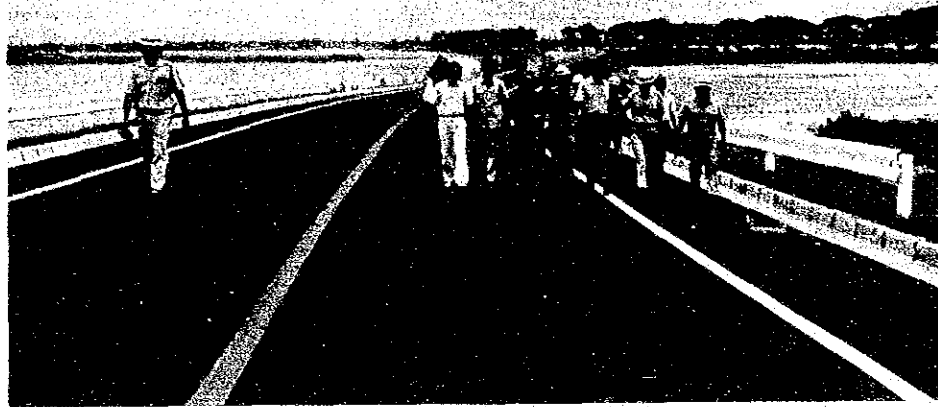
Meghna Bridge (Dhaka Side Approach Road)
