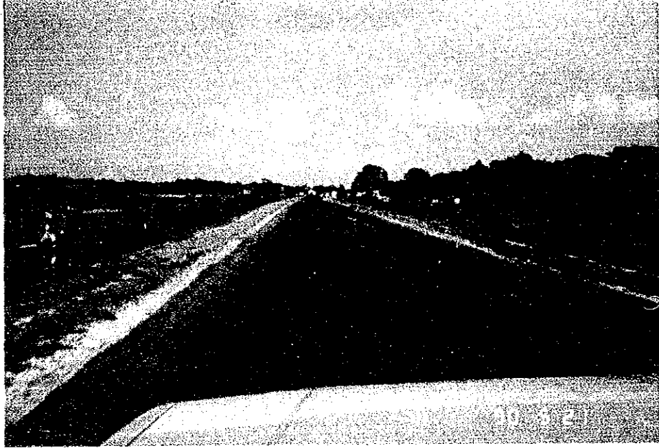
Dhaka - Chittagong National Road (Road Improvement is Completed in Chandina Bypass)
