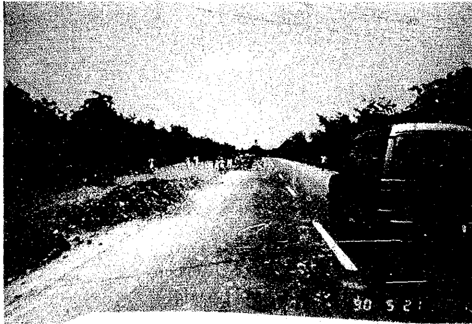
Dhaka - Chittagong National Road (Between Dhaka and Sitalakhya Bridge)
