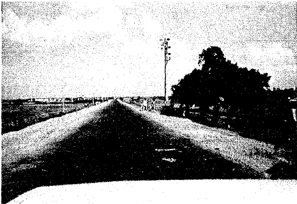
Dhaka - Chittagong National Road (Near the End of Approach Road at Comilla Side, Completion of Road Improvement is Scheduled in Mid 1991)
