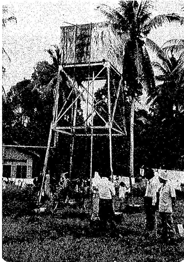
Elevated water tank
