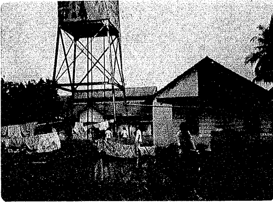
Elevated water tank & well pump house
