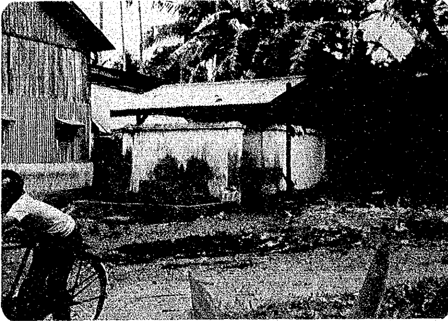
Artesian deep well constructed in Dutch age
