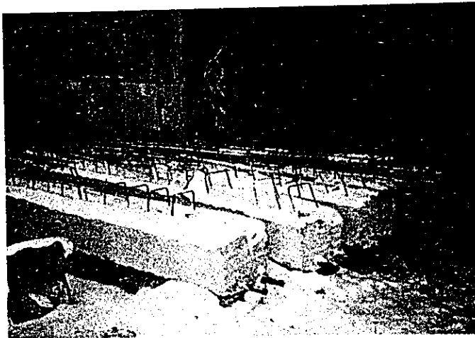
Photograph 1.6.11 Precast beam members left on construction site of RPC building, as in the previous photograph. A member covers one span. Top of the beam reinforcing bars is exposed at a portion where cast-in-place concrete is to be laid for connection with a floor panel. After assembling beam members, two main bars are provided at the two solid steel angle portion of the reinforcing bars, and then the main bars are welded, followed by placing of concrete. (Leninakan)
