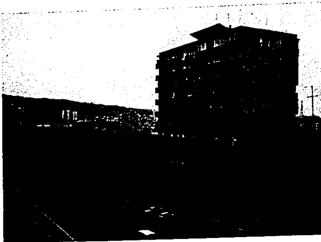
Photograph 1.6.1 Eleven-storied apartment house of framed precast reinforced concrete (RPC) construction and five-storied apartment houses of reinforced masonry (RMS) construction standing along the main street of capital Yerevan. (In most of the buildings in Armenia, purplish tuff is used as structural and exterior finishing material over the external faces.)
