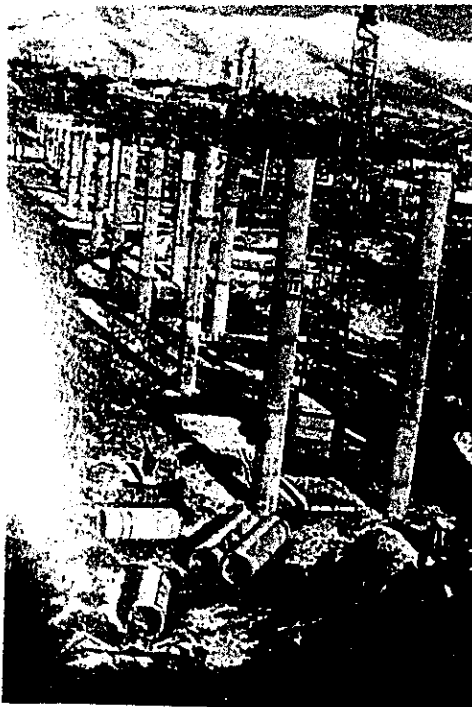
Photograph 3.2.5 Road Bridge under Construction
