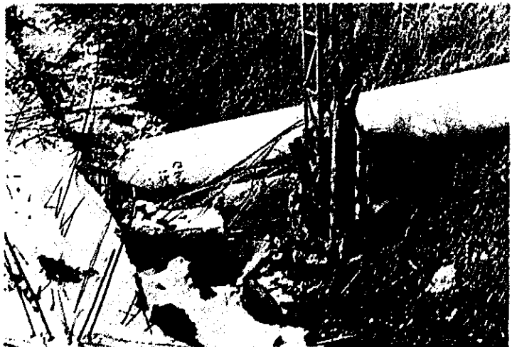
Photograph 3.2.19: Damaged Concrete Electric Pole and Temporary Restoration (Spitak)
