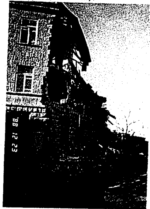
Photograph 3.1.36 Damaged gables at the second and third levels of a three-storied stone-built apartment house. The wall is of filled type, though apparently of masonry type, and the floor is of wood. It is unknown from where the long PC panel has dropped (Leninakan).
