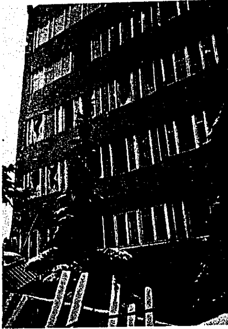
Photograph 3.1.69 When viewed at close range, many window-panes are broken and vertical members which appear to be reinforced concrete pillard suffered large cracks.
