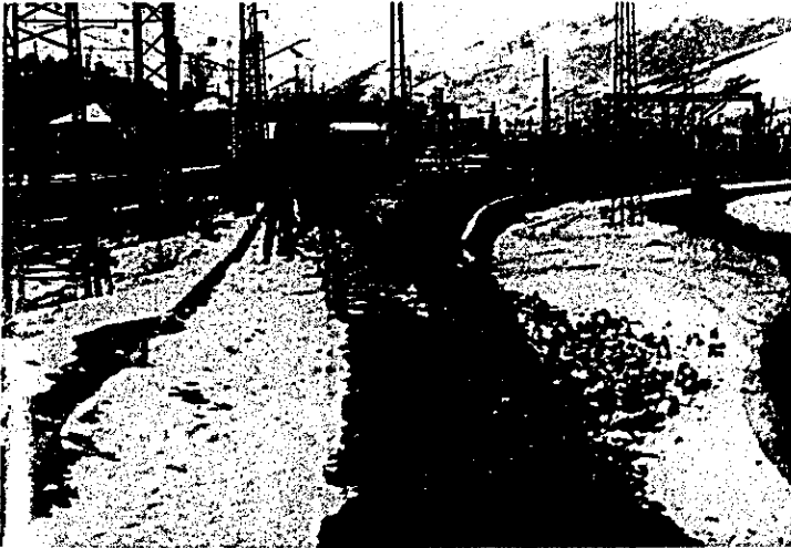
Photograph 3.2.17: Damaged Railroad (photographed by Soviet expert immediately after the earthquake)
