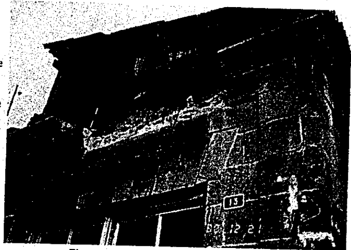
Photograph 3.1.36 Damaged gables at the second and third levels of a three-storied stone-built apartment house. The wall is of filled type, though apparently of masonry type, and the floor is of wood. It is unknown from where the long PC panel has dropped (Leninakan).
