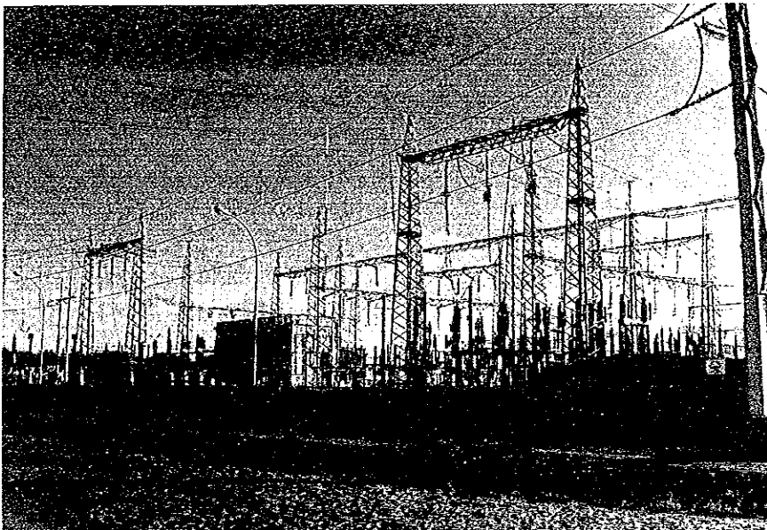
San Lorenzo Substation
