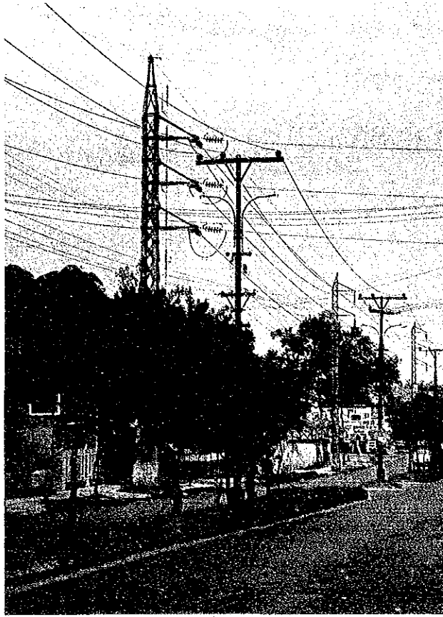
66 kV Transmission Line and 23 kV Distribution Line
