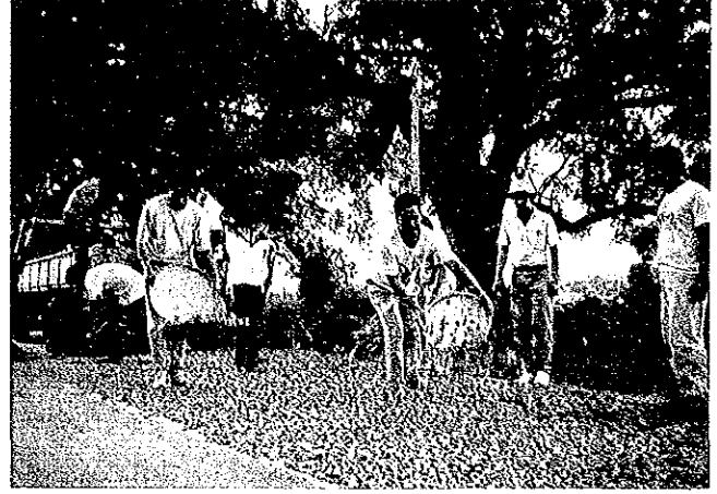
Bituminous penetration macadam, base layer aggregate spreading by hand
