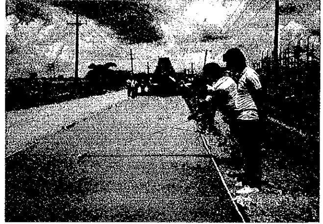
Finishing of cement concrete surface
