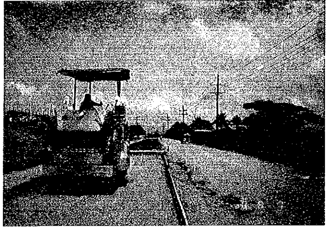
Compaction of trimmed subbase course
