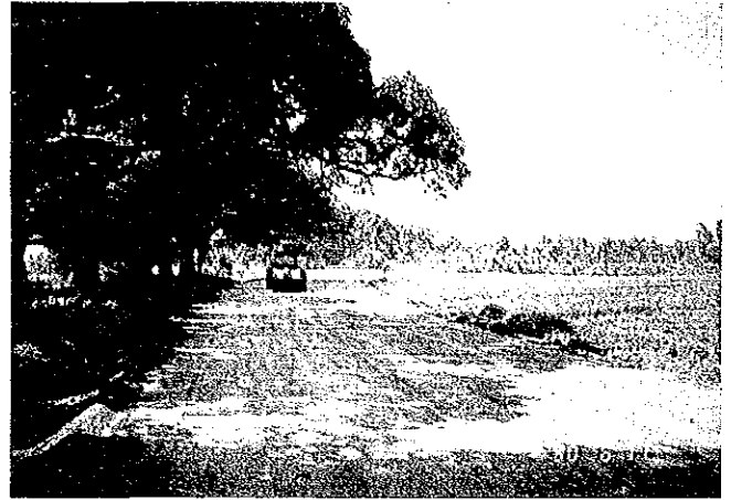
Compaction of subbase course materials
