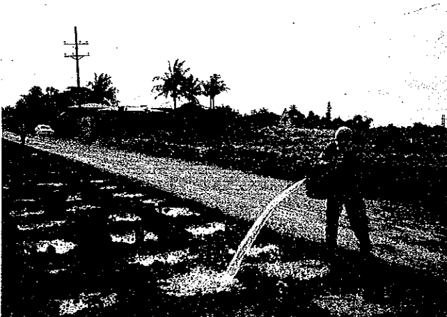
Water curing of hardened concrete
