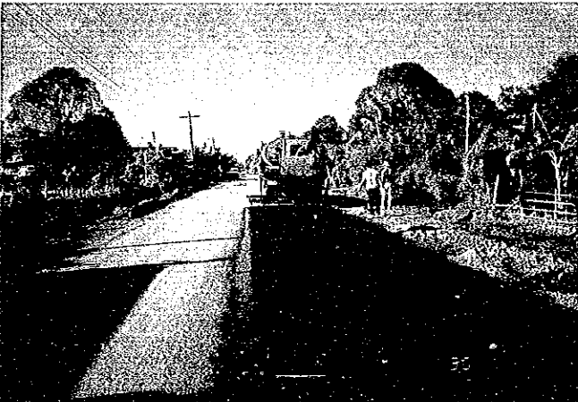
Double bituminous surface treatment, asphalt binder spraying by asphalt distributor
