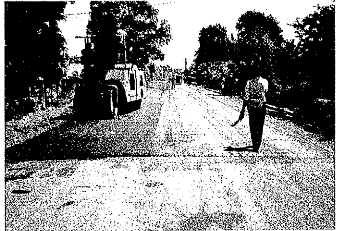
Rolling of asphalt concrete (left) and finished asphalt concrete surface course (right)
