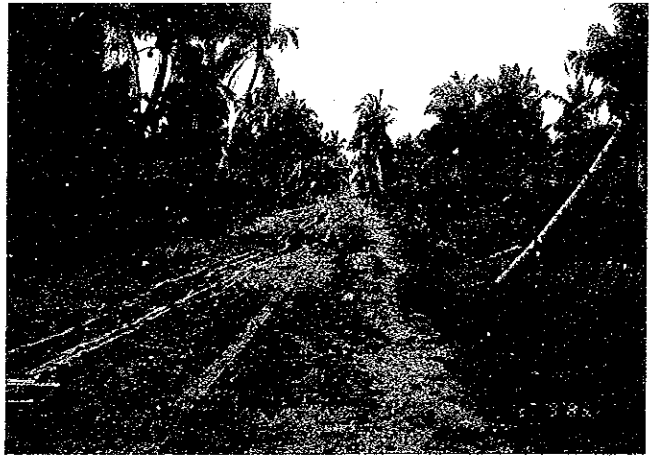
San Juanico-Sohoton Road, Samar Earth road
