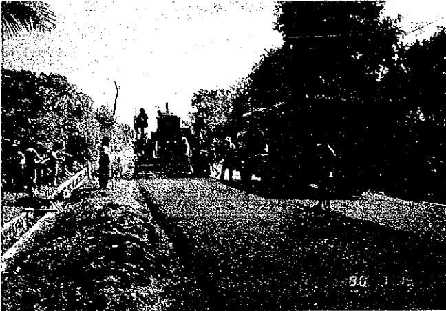
Laying of asphalt concrete by asphalt finisher
