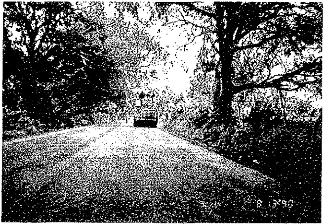
Finished bituminous penetration macadam (left) and stone layer rolling (right)
