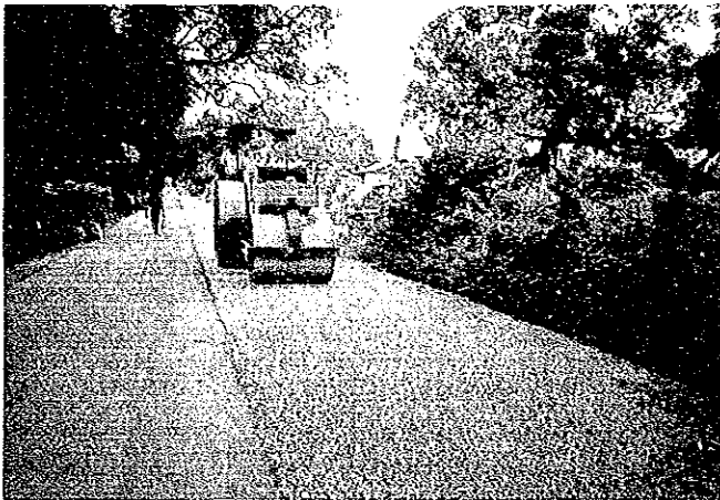
Bituminous penetration macadam, base layer compaction
