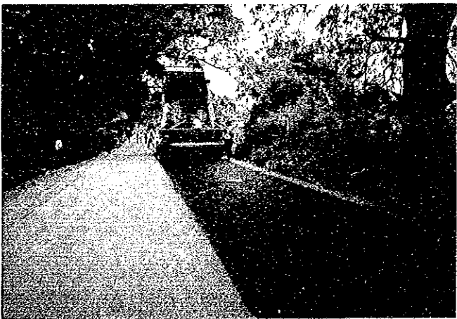
Bituminous penetration macadam, cover aggregate spreading
