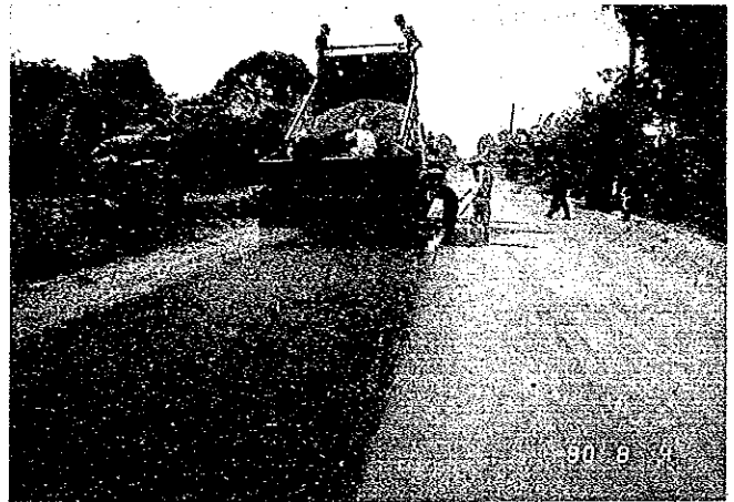
Double bituminous surface treatment, cover aggregate spreading by aggregate spreader
