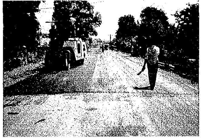
Rolling of asphalt concrete (left) and finished asphalt concrete surface course (right)
