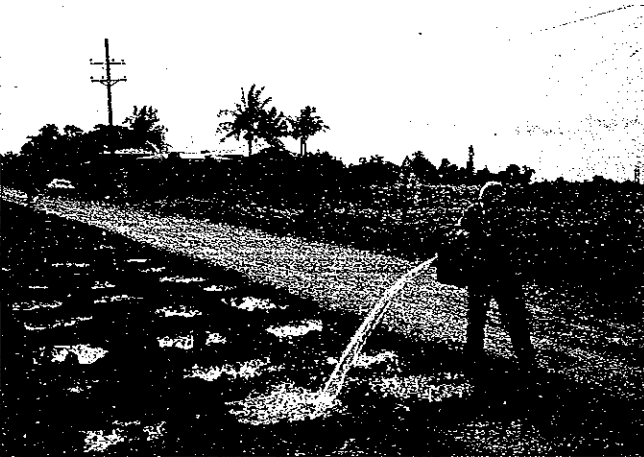
Water curing of hardened concrete
