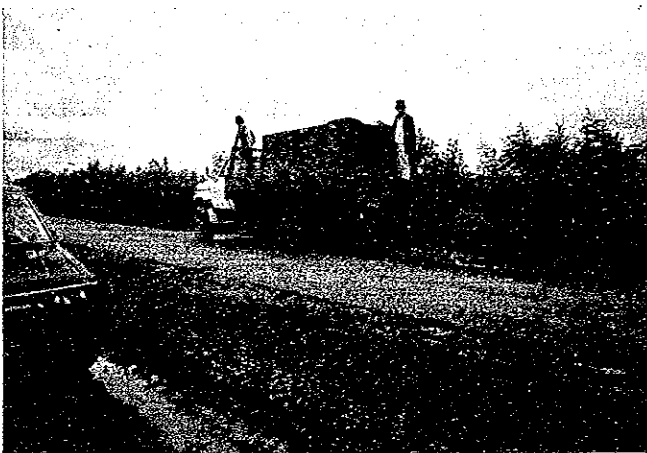
Watering of base course for compaction
