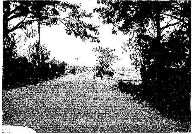
Bacnotan-Luna-Balaoan Road, I.a Union DBST pavement in fair condition
