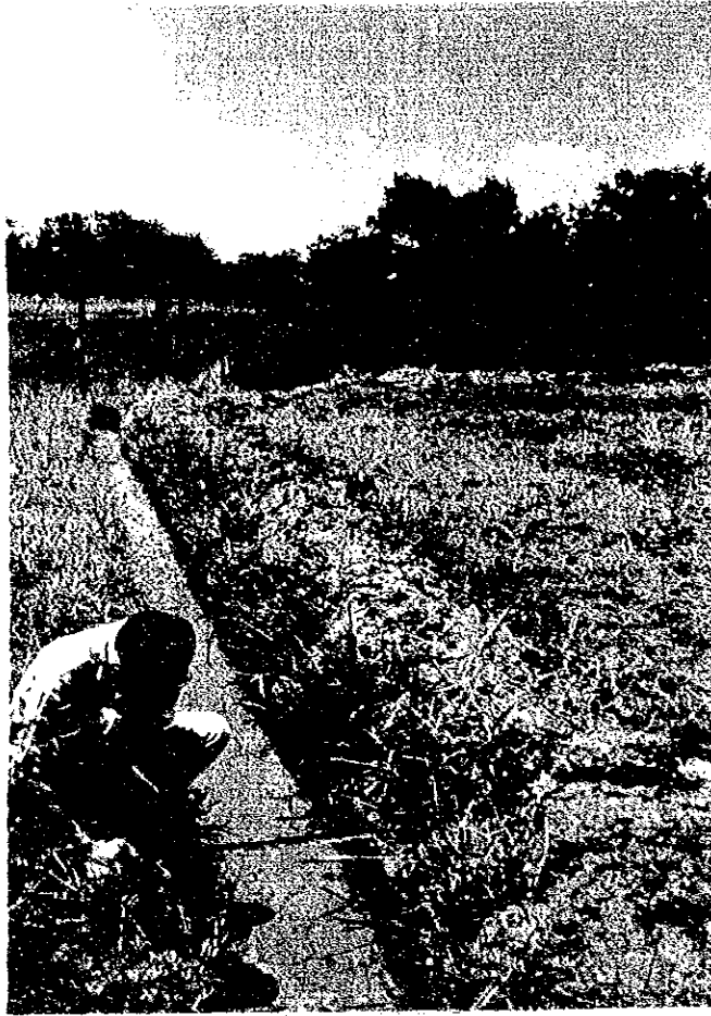
Existing Drainage Canal in the Central Research Station
