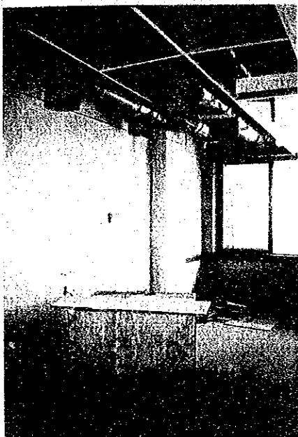
Exhaust Duct for Draft Chamber
