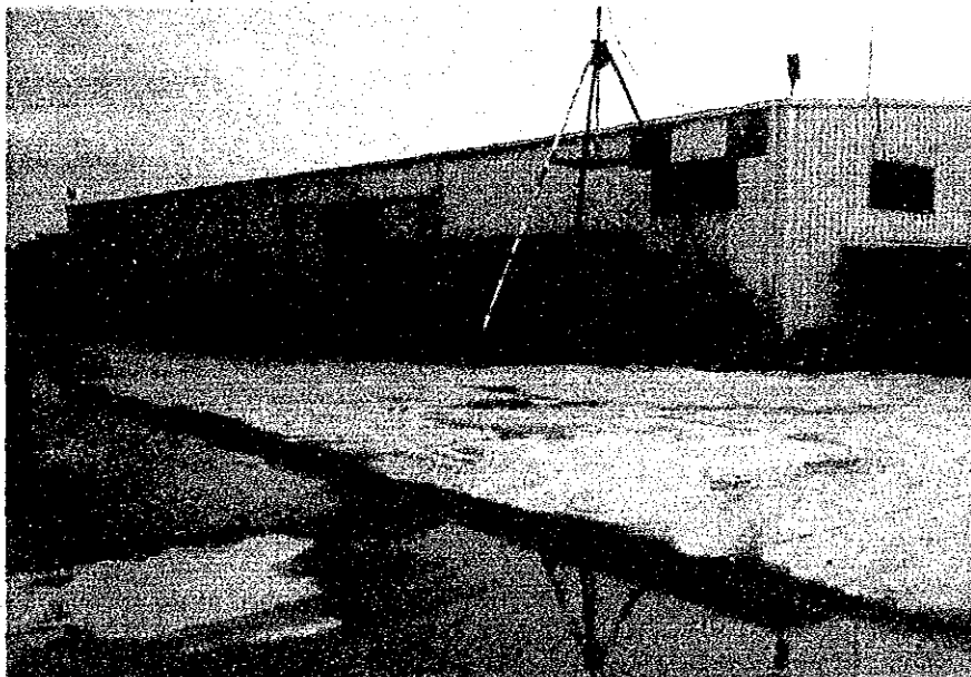
Existing Transit Shed
