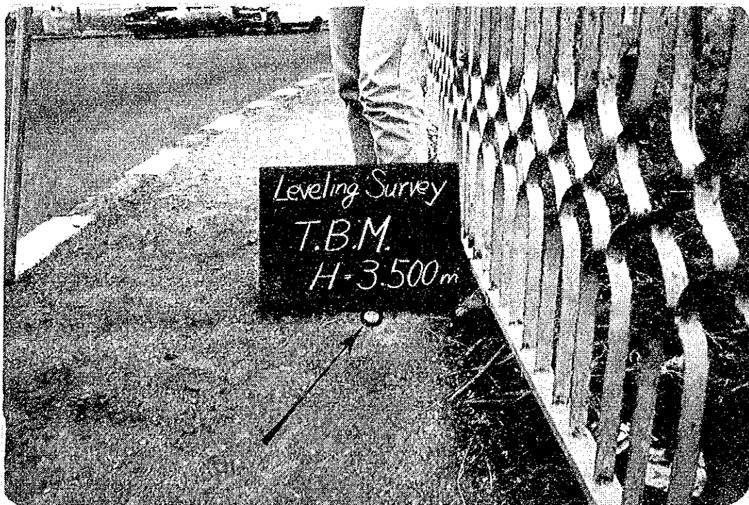
Photo B.6 Temporary BM in Khormaksar
