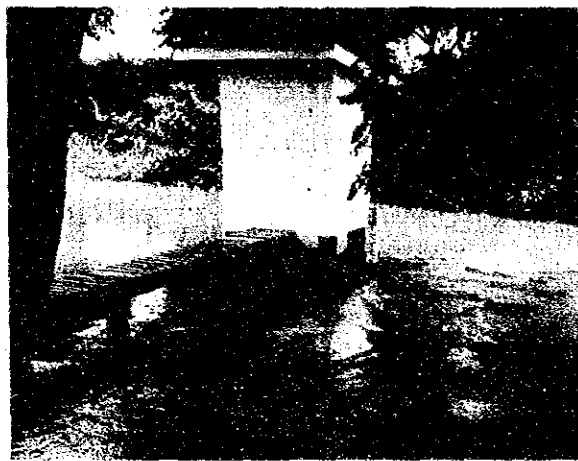
Automatic Water Level Gauge at Hong Xeng
