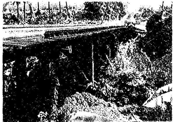
Existing : Timber Bridge : Substructures Reinforced Concrete
