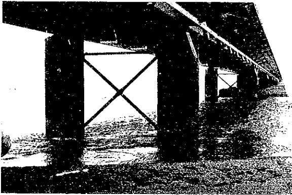
Pile bent piers supporting steel truss girder (Severe corrosion of the piers reported.)
