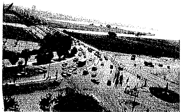
Omdurman side approach road to the existing bridge
