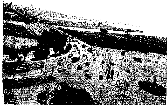
Omdurman side approach road to the existing bridge
