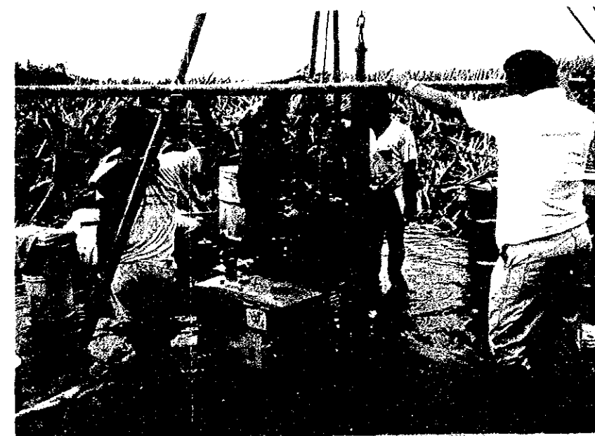
Boring works in Alika Swamp
