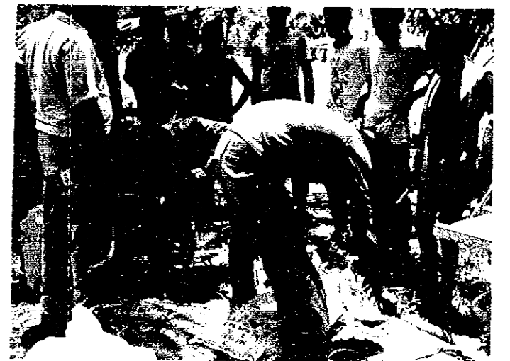
Installation of Concrete Monument of GPS Point
