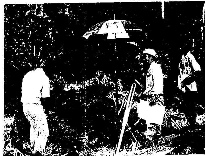
Road Centerline Survey
