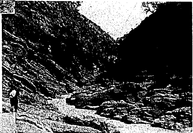
PHOTO-16 San Jacinto Project, dam site
