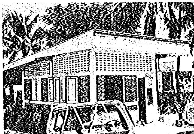
Telephone Office in San Patong District
