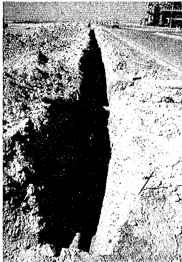
Pipeline of non-sterilized seawater (underground)
