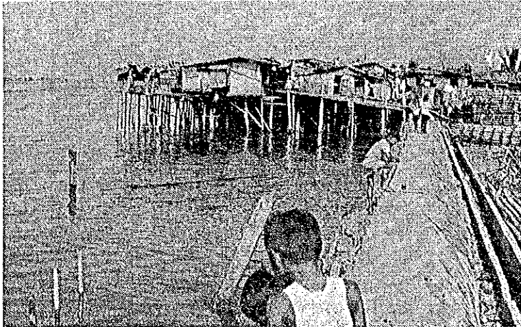
Housing Fixed on Water and Revetment (NAVOTAS)
