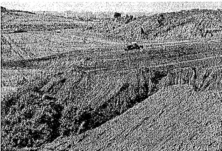
Artificially Deformed Land (Under Construc- tion)
