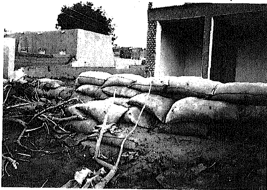
TEMPORARY BARRIER (MADE BY SAND BAGS) FOR FLOOD PROTECTION AT HOSH BANAGA VILLAGE, SHANDI
