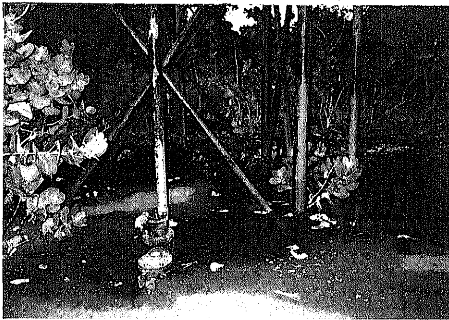
EXISTING WATER YARD INSTALLED AT HOSH BANAGA VILLAGE, SHANDI BURIED BASE OF ELEVATED TANK DUE TO INFLOW OF SAND CAUSED BY FLOODING OF THE NILE
