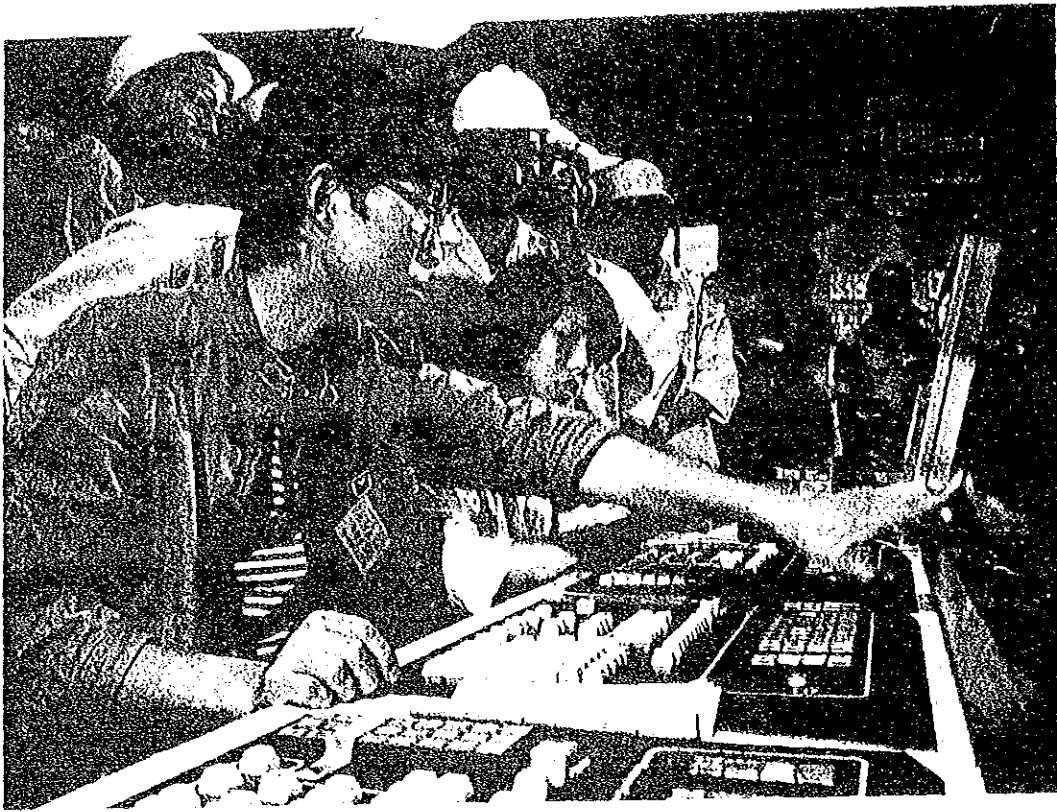
扬子30万吨乙烯中心控制室、投油试车 Control room in Yangzi 300,000 ton ethylene plant in trial running.
