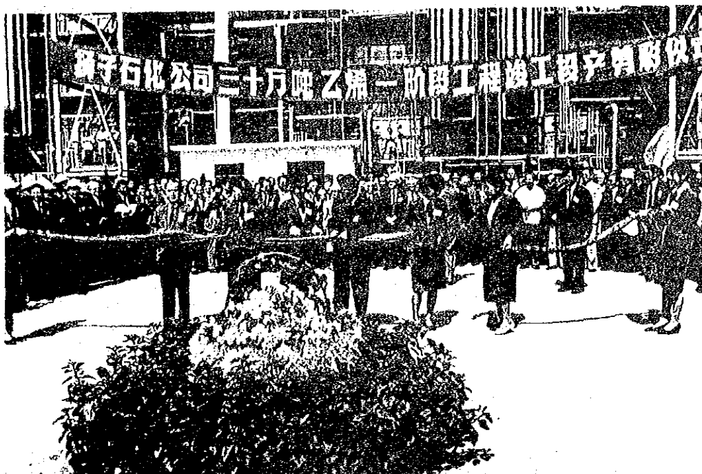
国务委员康世恩为扬子30万吨乙烯一期工程投产剪彩 State Council member Kang Si En cut the ribbon at the celebration of going into operation of the first phase of Yangzi 300,000 ton ethylene plant.
