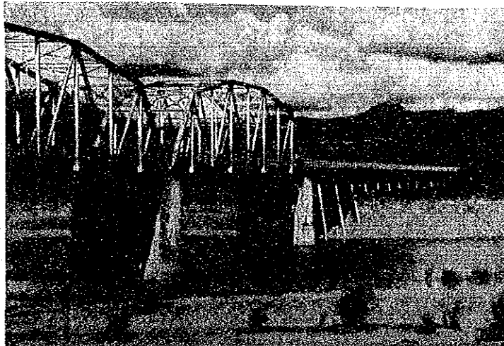
VIEW OF APPROACH BRIDGE
