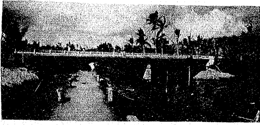
GENERAL VIEW OF GUINOBATAN BRIDGE
