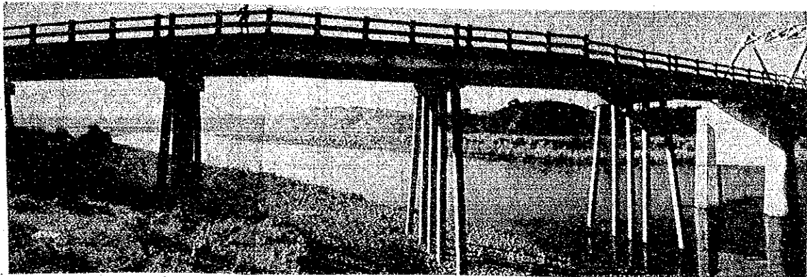
GENERAL VIEW OF PINACANAUAN BRIDGE
