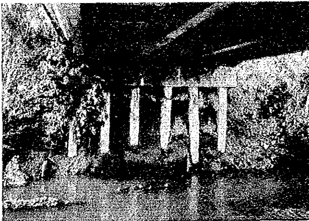
EXPOSED ABUTMENT AFTER WASHING AWAY OF SLOPE PROTECTION
