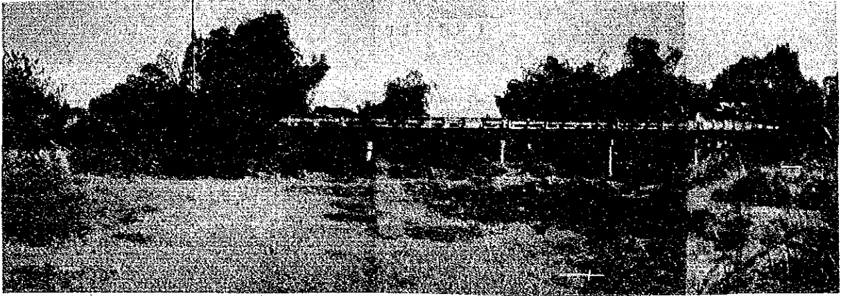
GENERAL VIEW OF SAN ROQUE BRIDGE
