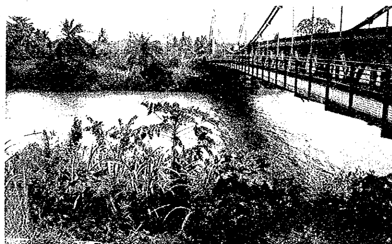
PROPOSED BRIDGE SITE DOWNSTREAM OF EXISTING BRIDGE FROM ACCRA SIDE
