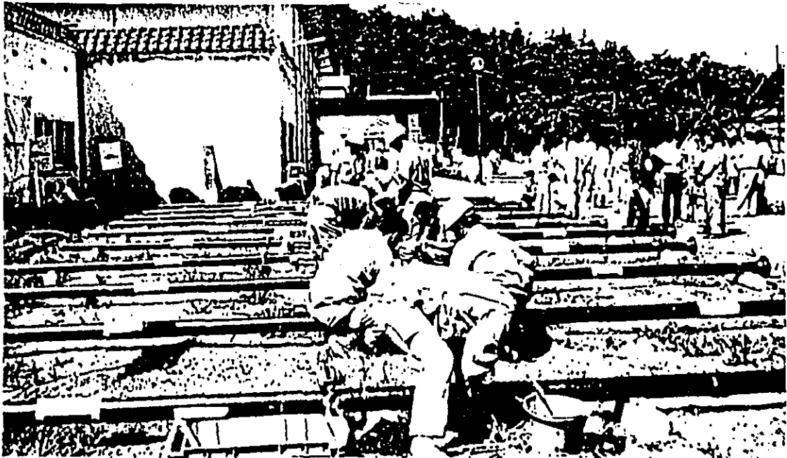
Figure-12. Training Course of pipe laying held by Small Water Supply Association
