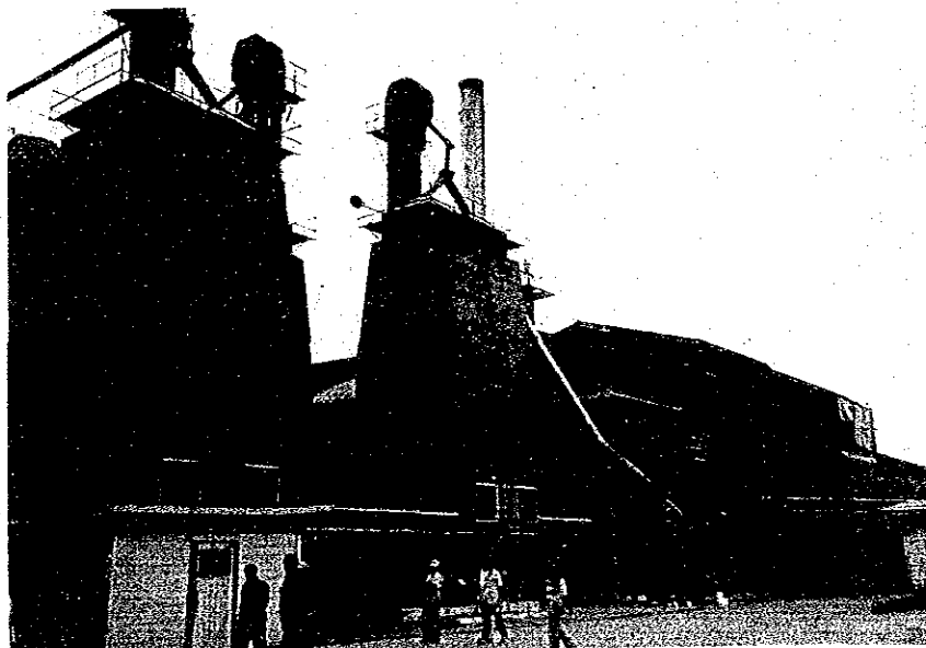
3. Parboiled Rice Plant ... Presently under repairing.
