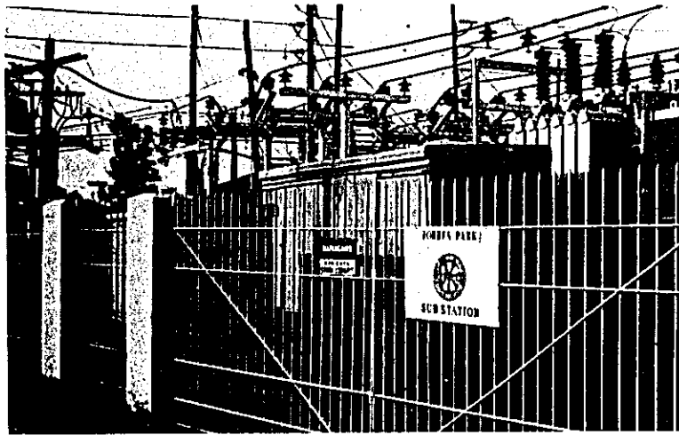
69KV Metal-clad Substation at Manila
