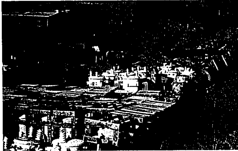
Stock of Pole Transformer at CAGELCO
