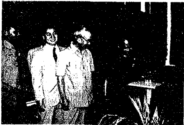
Switch-on of operations at Banko coal gasification test plant by Minister B.J. Habibie and Ambassador T. Muto (1987)
