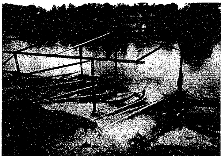
Fig. 10-1-8 Pictures Related to Rivers and Bridges (A - K)
