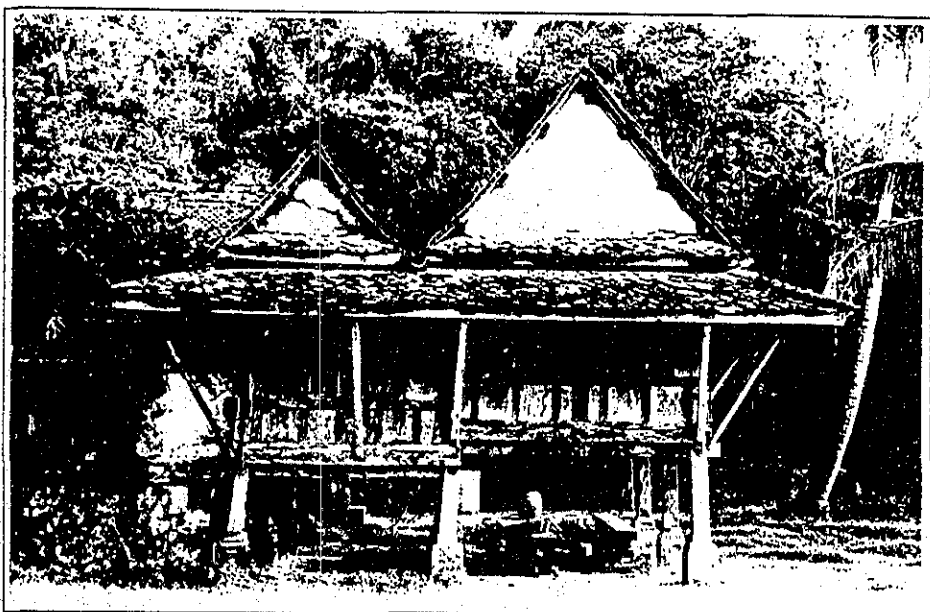
Traditional Thai Residence in Southern Thailand, Songkla Province
