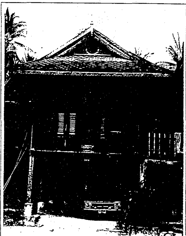
Typical Southern Residence, Yala Province
